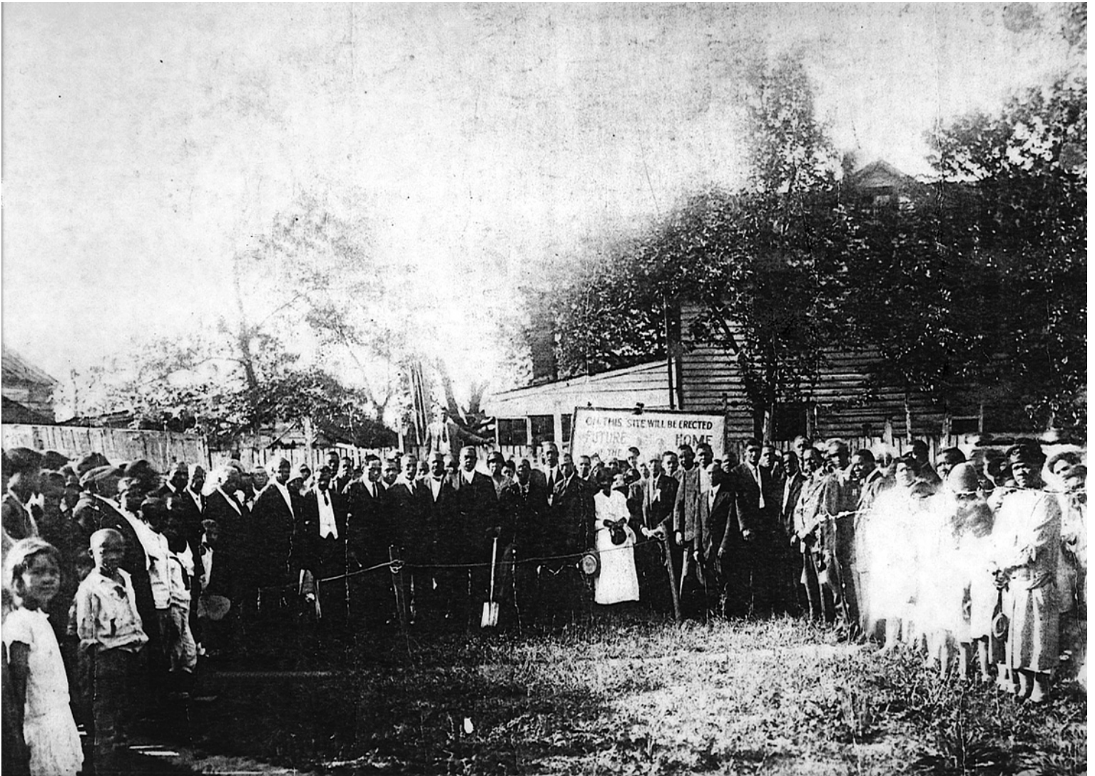
Deanwood residents at the groundbreaking for First Baptist Church of Deanwood's second building in 1909. Photo courtesy of Elaine Bowman.
